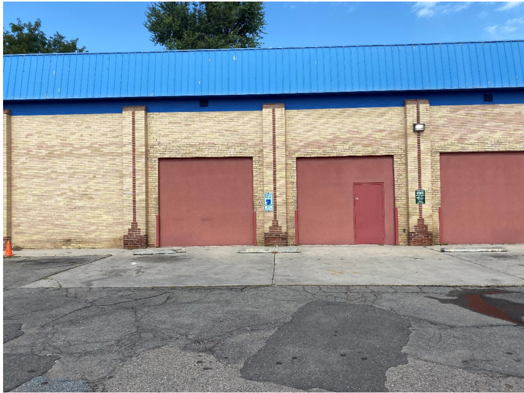
Photo 1- Facing north looking at the building façade that faces Longs Peak Avenue. Blight factors present include, deteriorated façade, roof and loading areas, deterioration of parking surface, inadequate parking striping.
