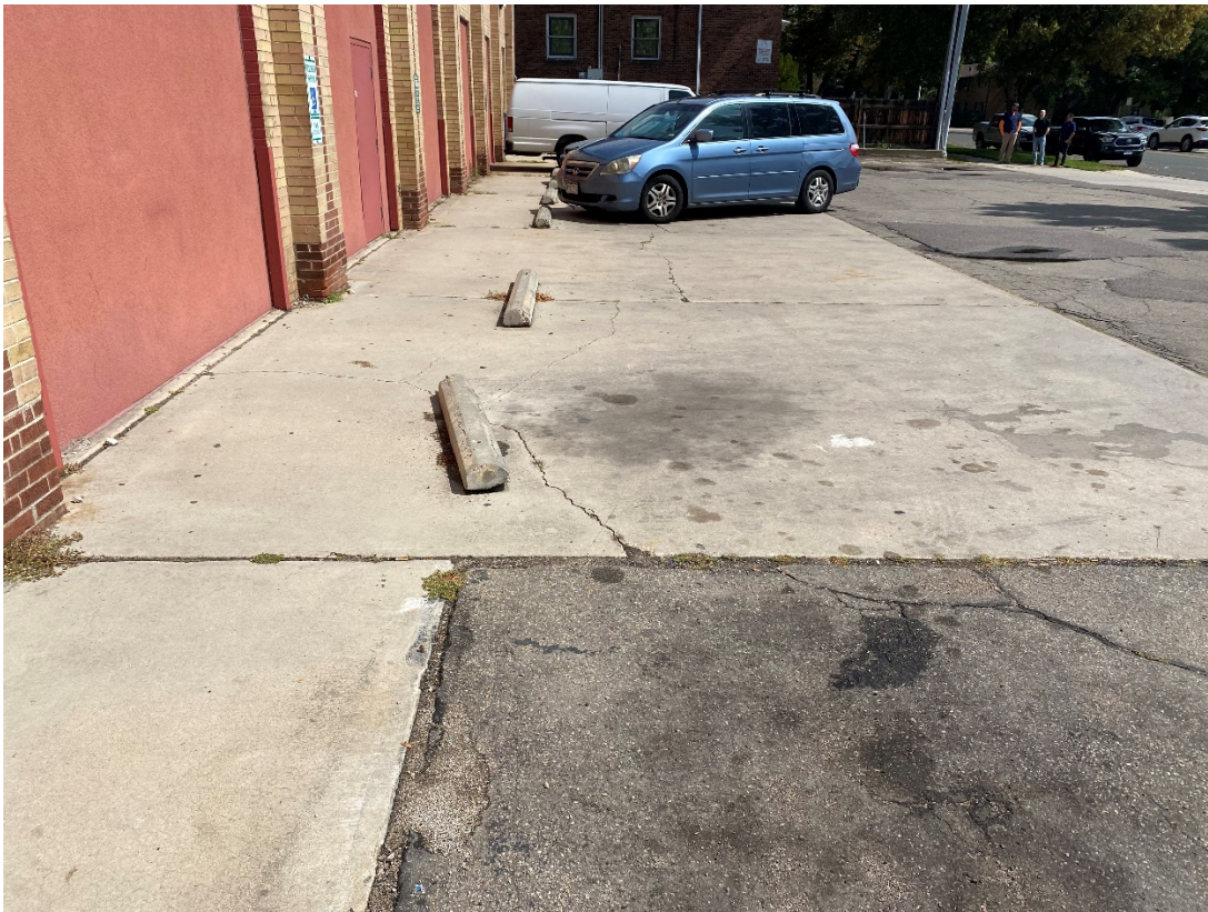
Pic 4- Looking east at the parking lot on the site. Inadequate striping, un-maintained parking surface, trash and poor drainage are all factors present at this site.
