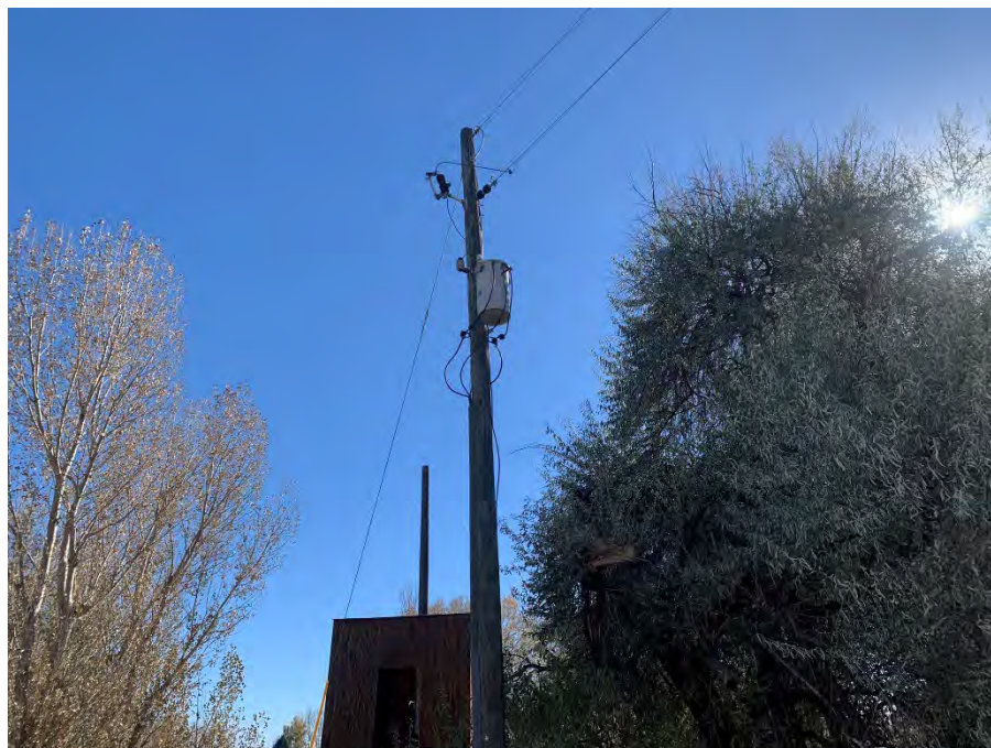
Photograph 6: Pole-mounted transformer located on the northeast corner of the site.
