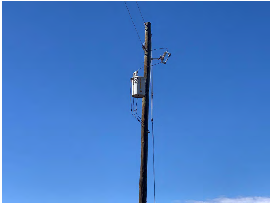
Photograph 34: Pole-mounted transformer located on the northwest portion of the site.
